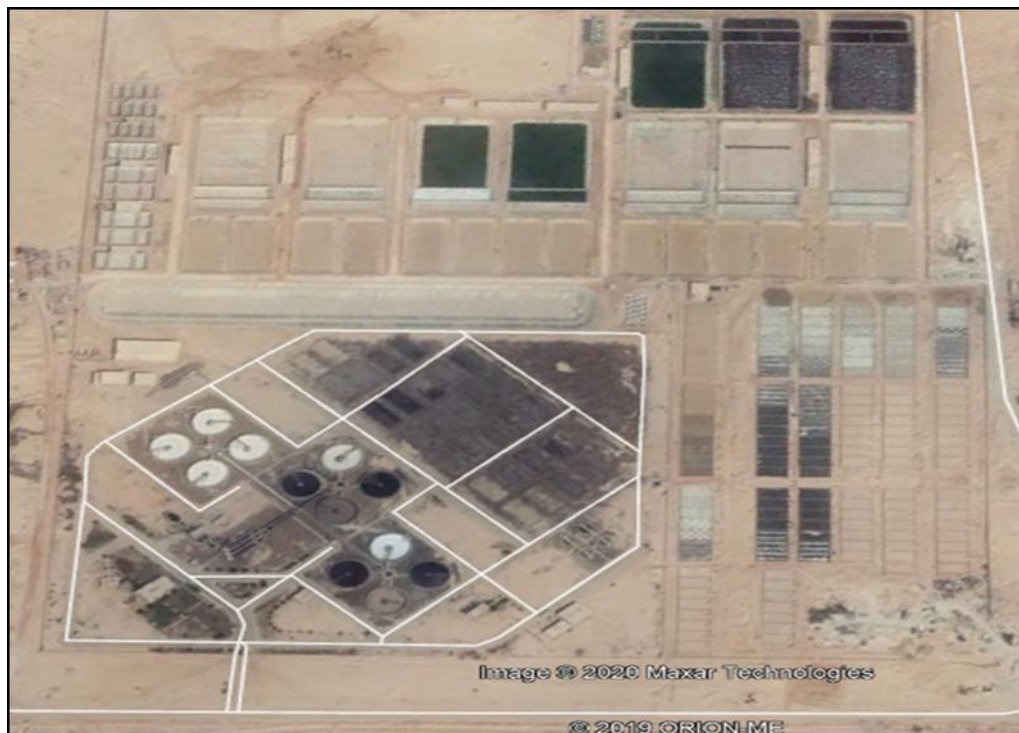
Fig. 1: The 10 th of Ramadan WWTP in (a) a general layout, (b) an adapted photo from Google earth, (February, 2020)
