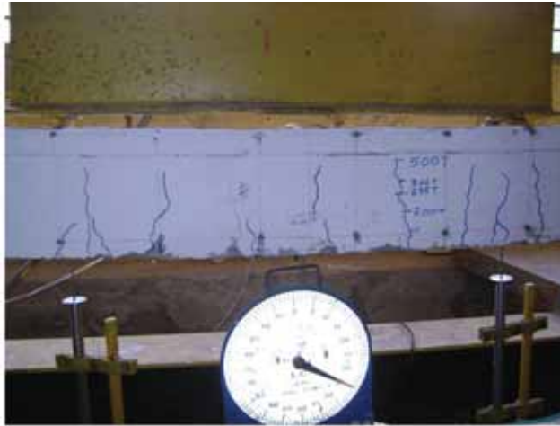
Fig. 9: Typical crack pattern of a perfect beam
