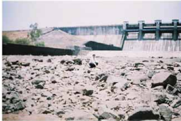
Fig. 1: Photograph showing riprap in the tail channel portion of Pawana dam spillway
