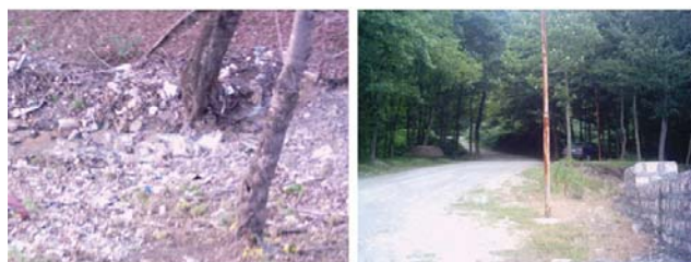
Fig. 3: Access road to the site and the high seepage flow of 10-20 liters per second observed.
