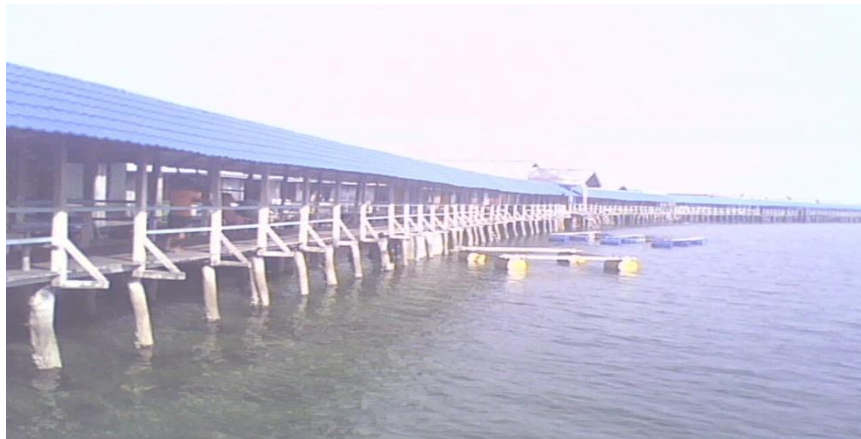
Fig. 1: The Bajo tribe settlements on the sea surface. There are about 250 stilt houses arranged in U formation that is occupied about 1,400 inhabitants. To connect all the houses, built corridors of wooden bridges around the entire village along 4,000 meters.
